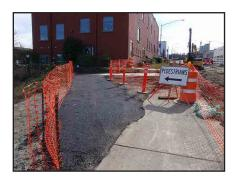
During construction, pedestrians should be re-routed on an accessible path; Source:SoundTransit
