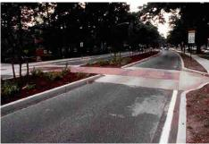
Speed Hump (top); Speed Table (bottom); Source: PBIC
