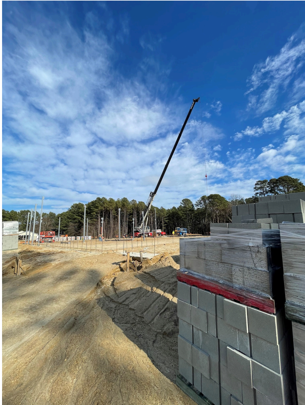
Hodge Road Fire Station Construction
