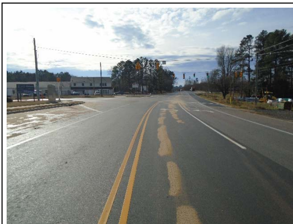
Looking south along Hodge Road at Spectrum Drive intersection
