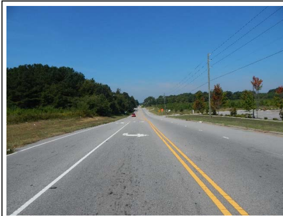
Looking east along Poole Road from the Hodge Road intersection
