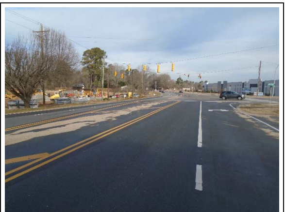
Looking north along Hodge Road at Spectrum Drive intersection
