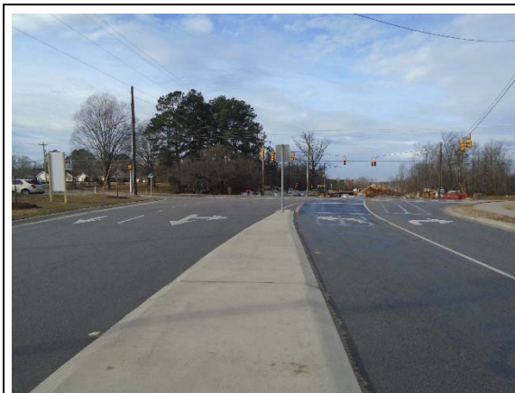
Looking west along Spectrum Drive at Hodge Road intersection
