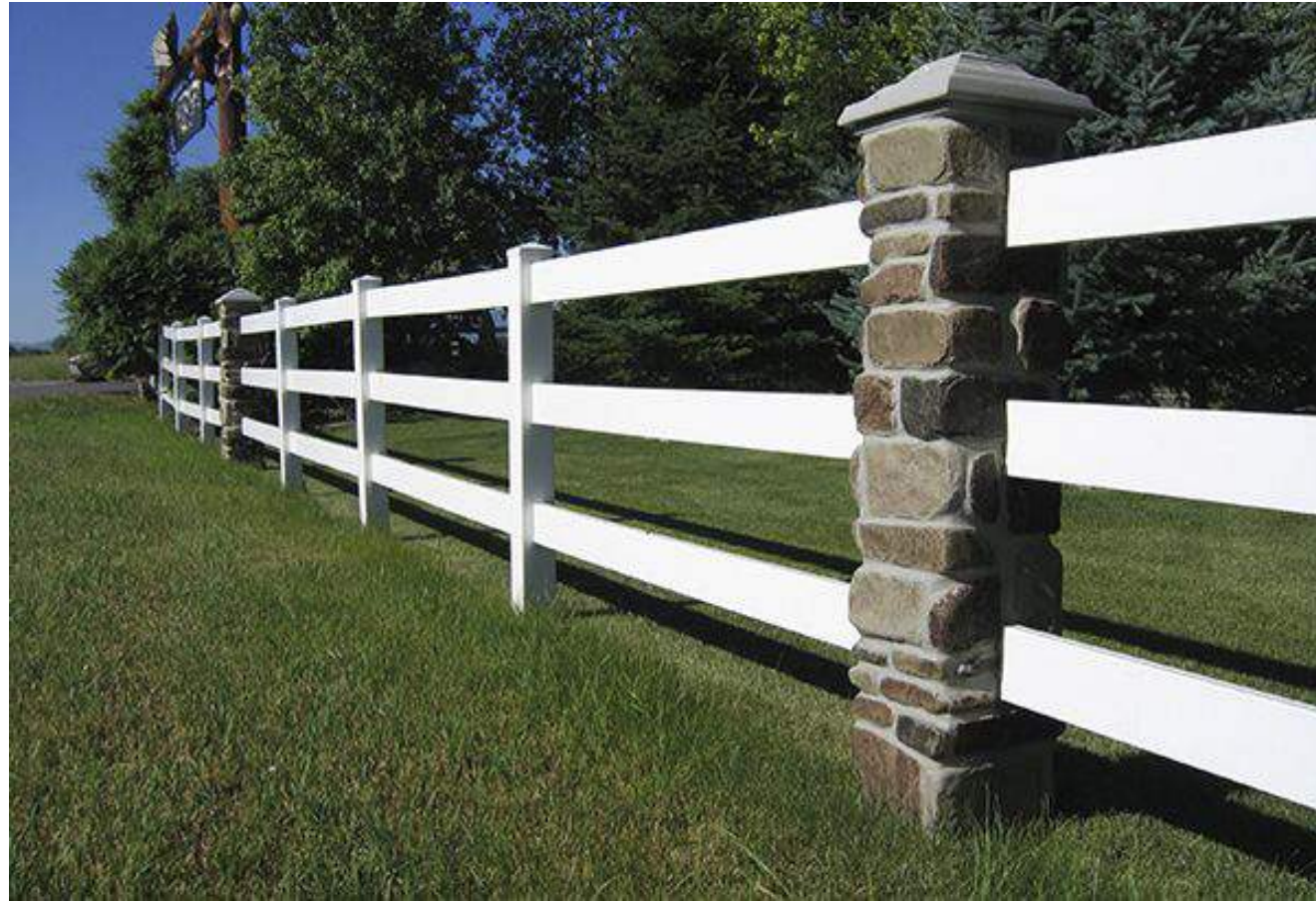
WHITE SPLIT-RAIL FENCE WITH MASONRY COLUMNS EVERY 50'
