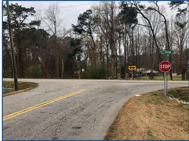
Westbound Approach of Lynnwood Road at Hodge Road
