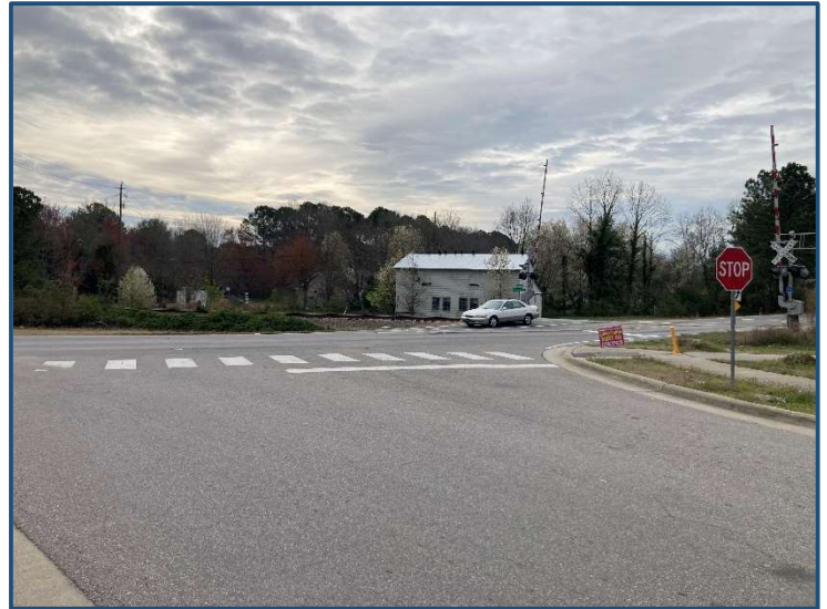
Eastbound Approach of Crosstie Street at Bethlehem Road/First Avenue Road
