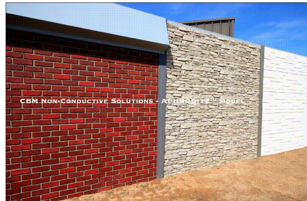
TYPICAL MASONRY WALL OPTIONS
