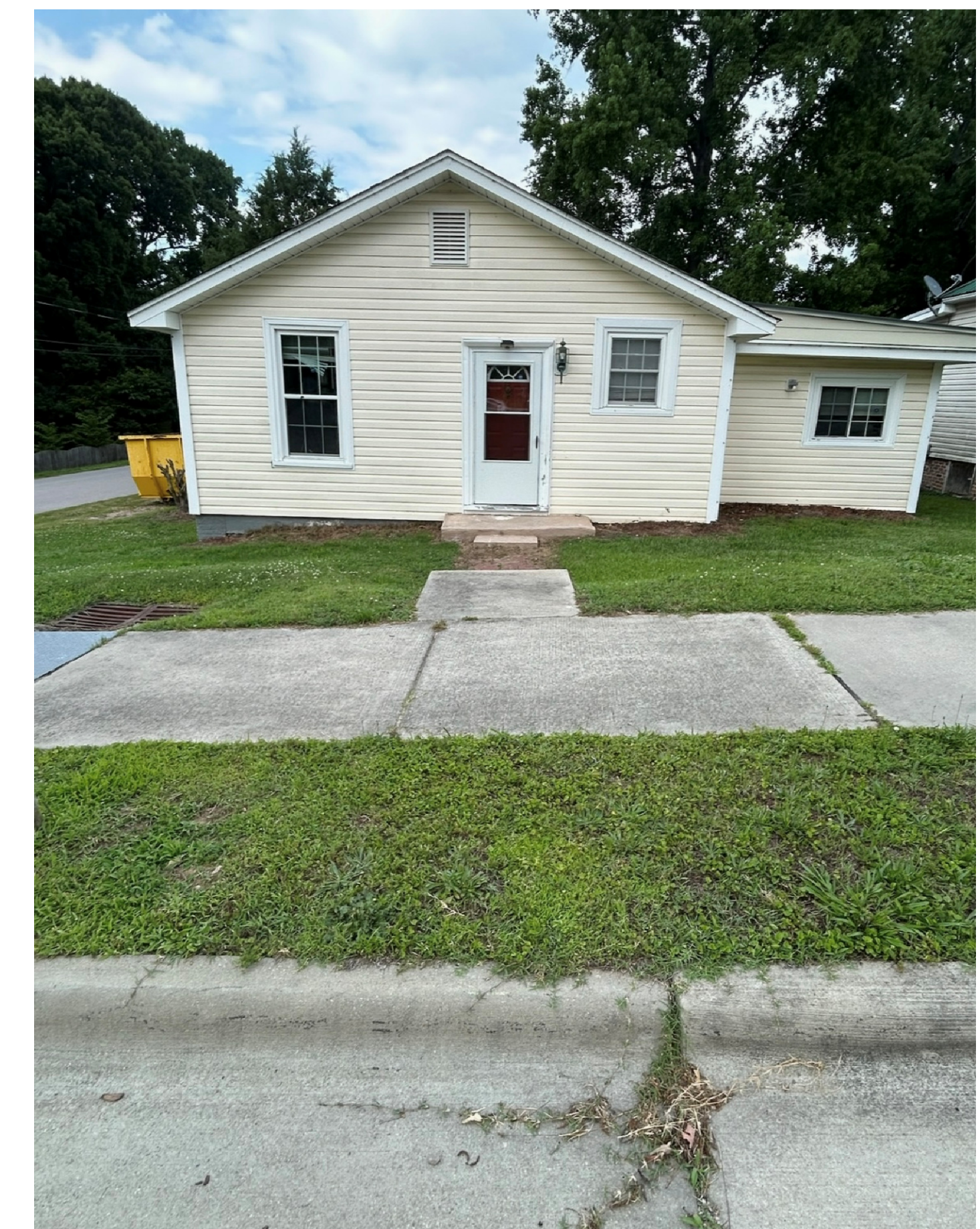
EXISTING VINYL SIDING
