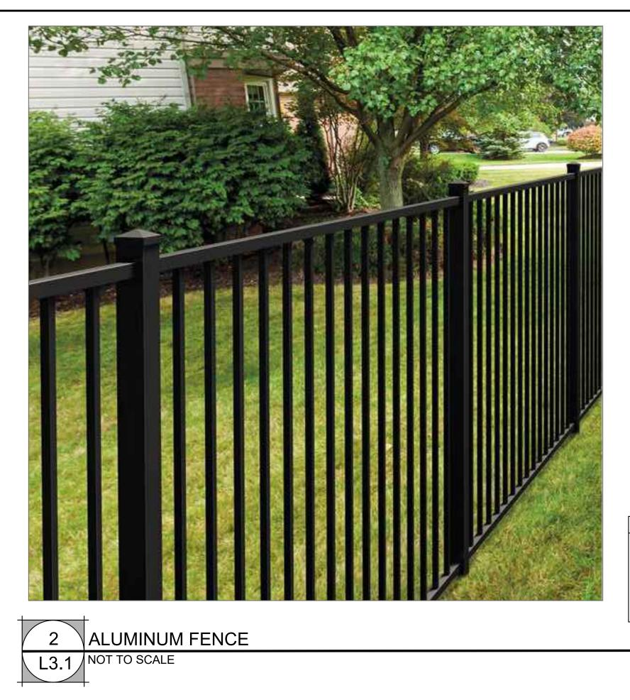
ALUMINUM FENCE REQUIREMENTS STYLE: 2 RAIL MATERIAL: ALUMINUM MATERIAL: ALUMINUM HEIGHT: 4' COLOR: BLACK NOTE: OWNER TO APPROVE FENCE PRIOR TO ORDERING. FENCE FOOTING TO BE DESIGNED PER MANUFACTURER'S SPECIFICATIONS.
