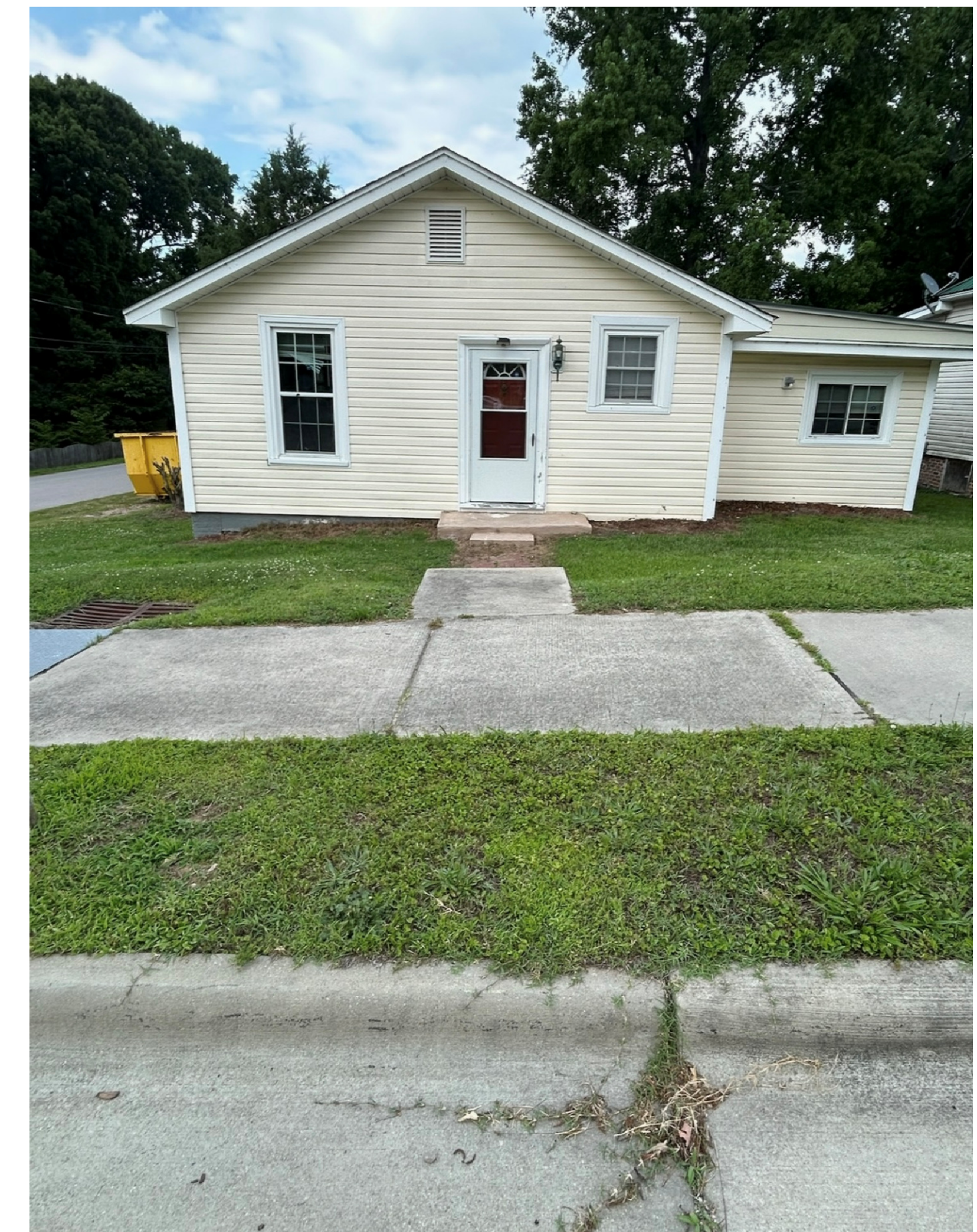
EXISTING VINYL SIDING
